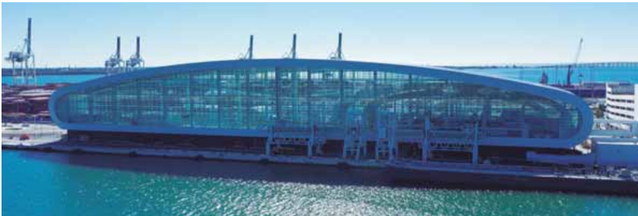
NORWEGIAN CRUISE LINE - TERMINAL B, FLORIDA ARQUITECTO: BA. BERMELO AJAMIL & PARTNERS CONSTRUCTOR: THE OHIO STATE UNIVERSITY
